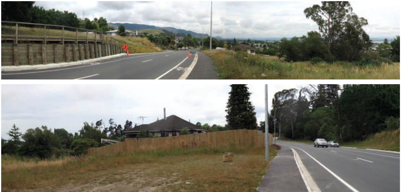
Figure2: Monitoring site at the start of the project, with positions to be monitored above and below the road
